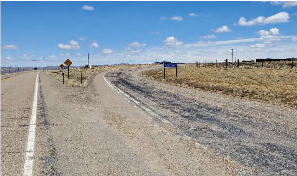
General Site Photo 14: Terminal Rd at SH370, looking Northeast
