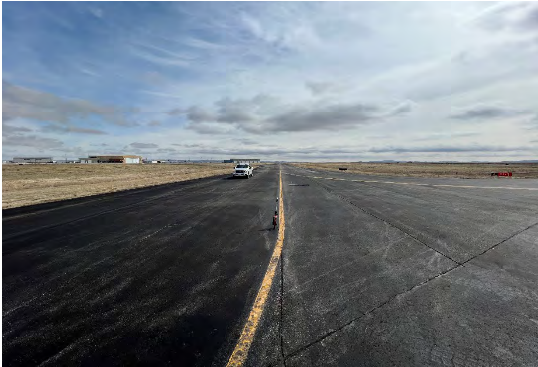
General Site Photo 11: Taxiway D at Taxiway A, looking Northeast
