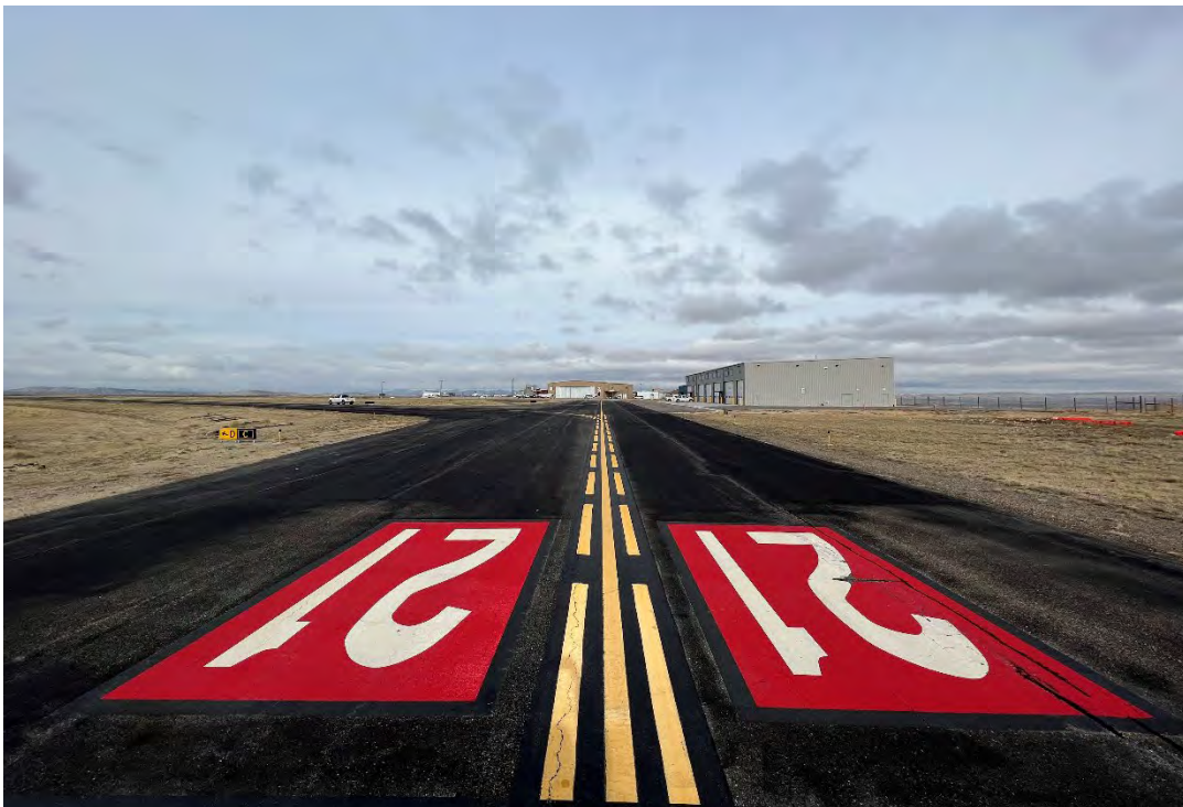
General Site Photo 10: Taxiway C at the Runway 3/21 Hold Line, Looking Northwest
