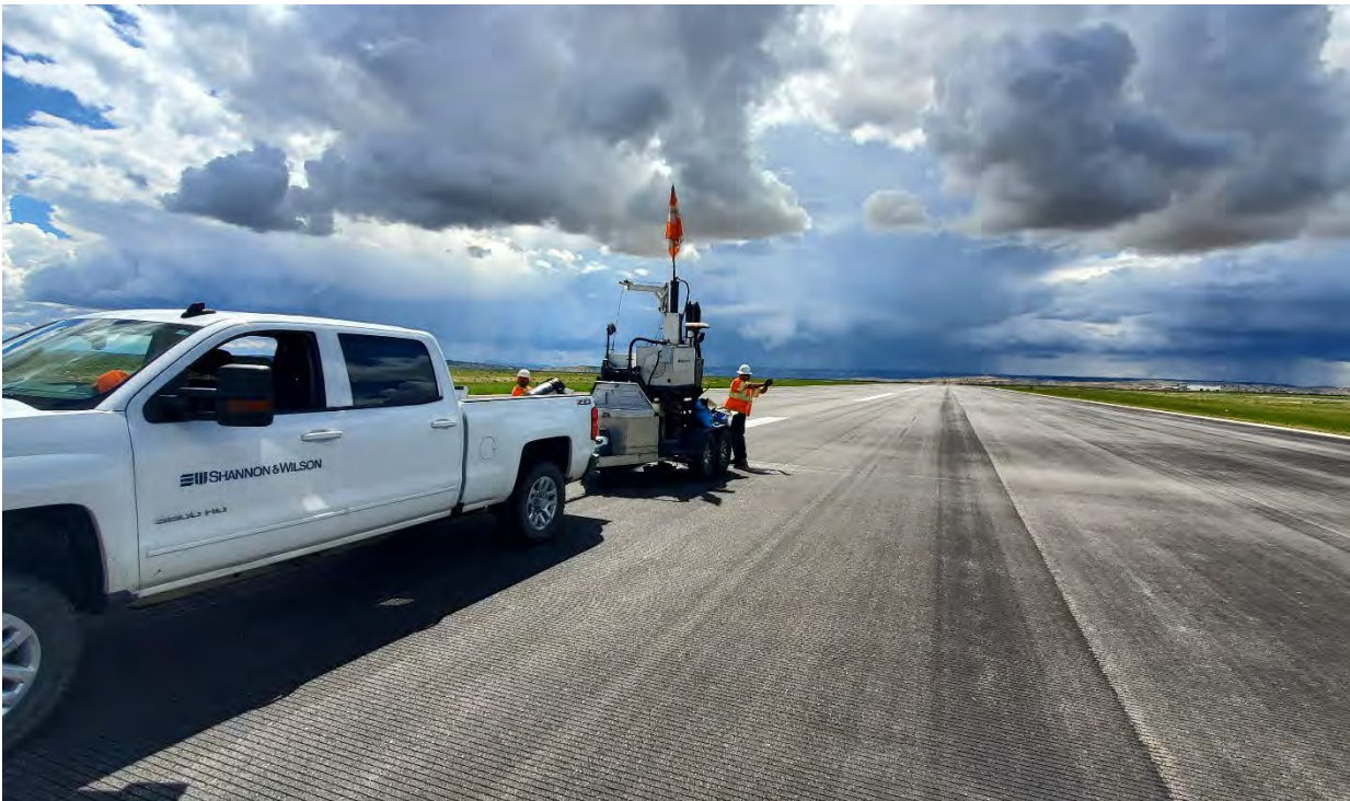
General Site Photo 2: S&W Drilling on Runway 9/27, looking West
