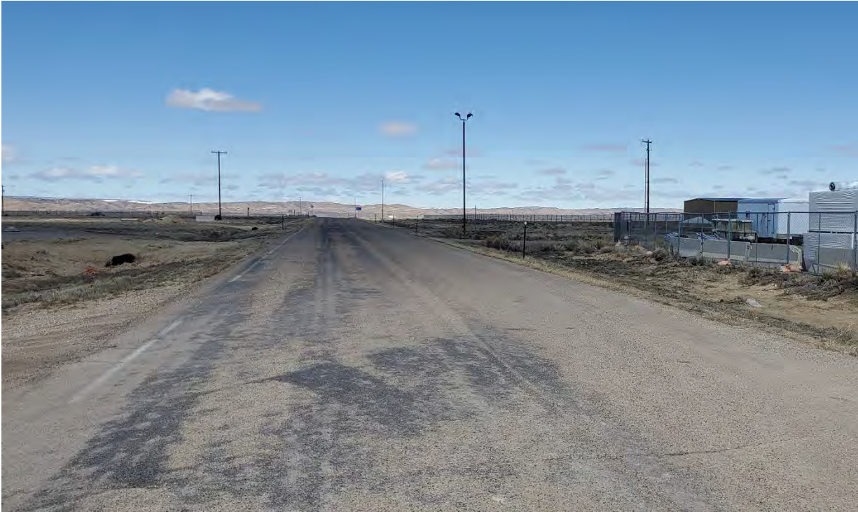
General Site Photo 15: Runway 9/27 at Runway 3/21, looking Northwest
