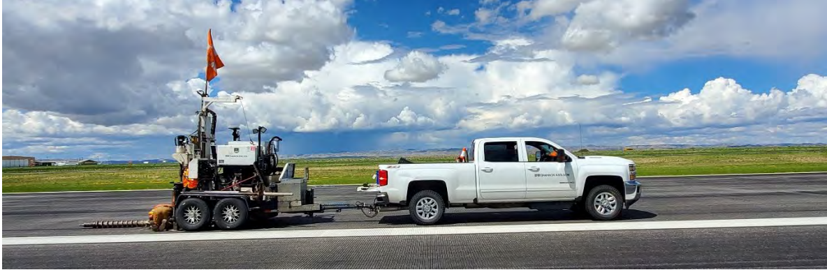
Figure 2-8: Pavement Drilling on Runway 9/27
