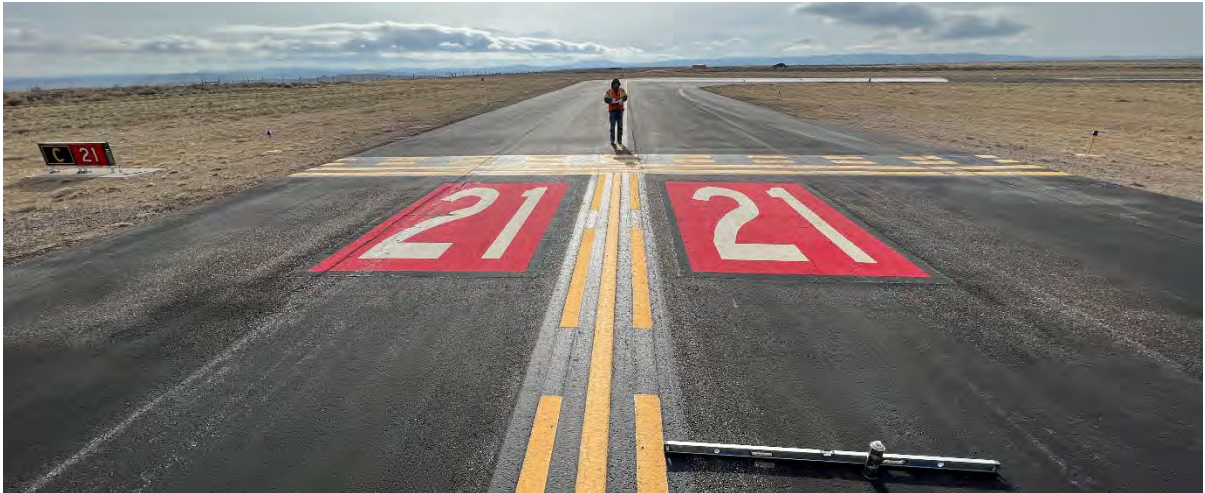
Figure 2-3: PCI Survey Being Conducted on Runway 3/21
