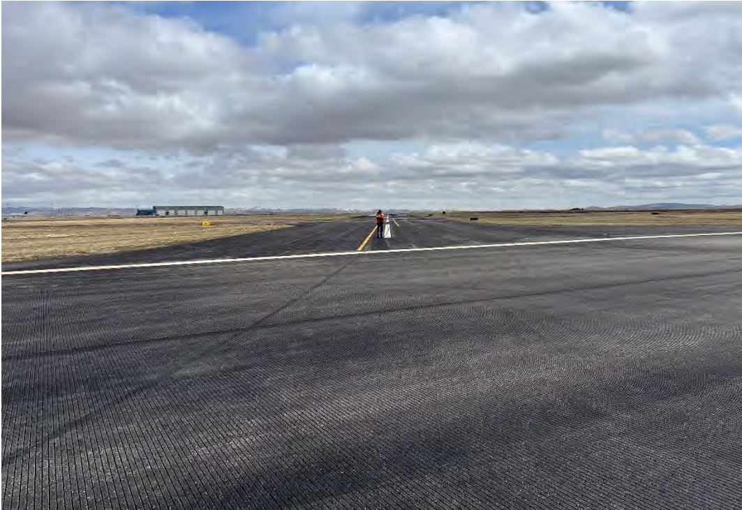
General Site Photo 7: Runway 3/21 at Runway 9/27, Looking Northeast
