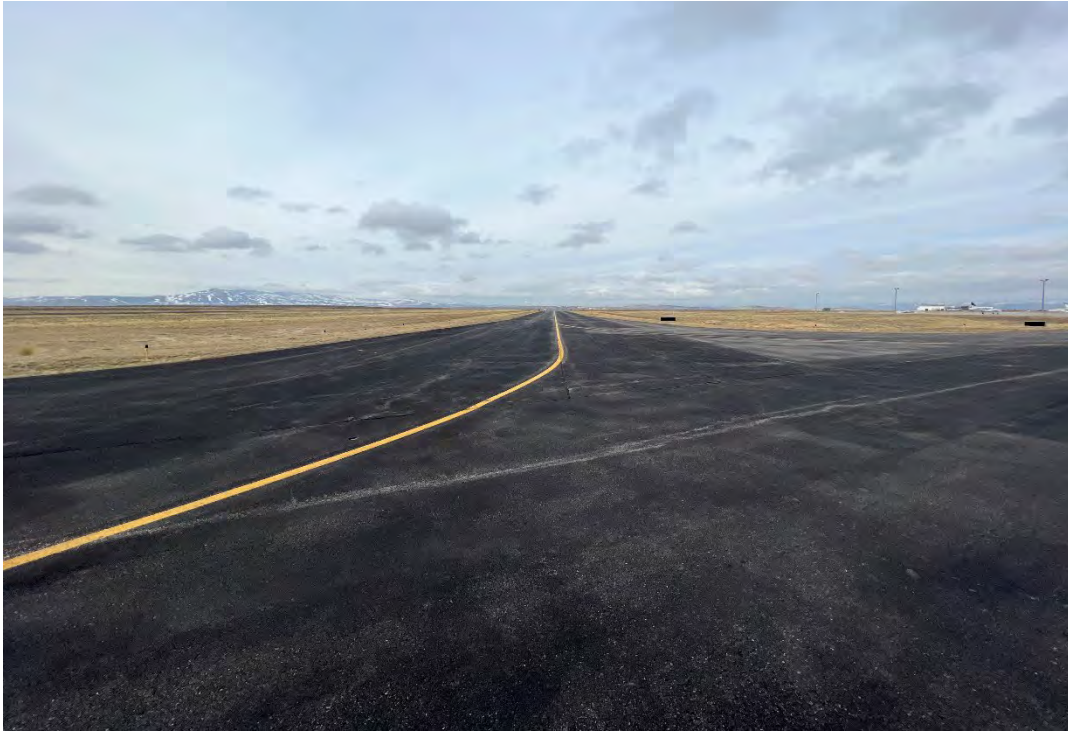
General Site Photo 13: Taxiway D at Taxiway C, looking Southwest
