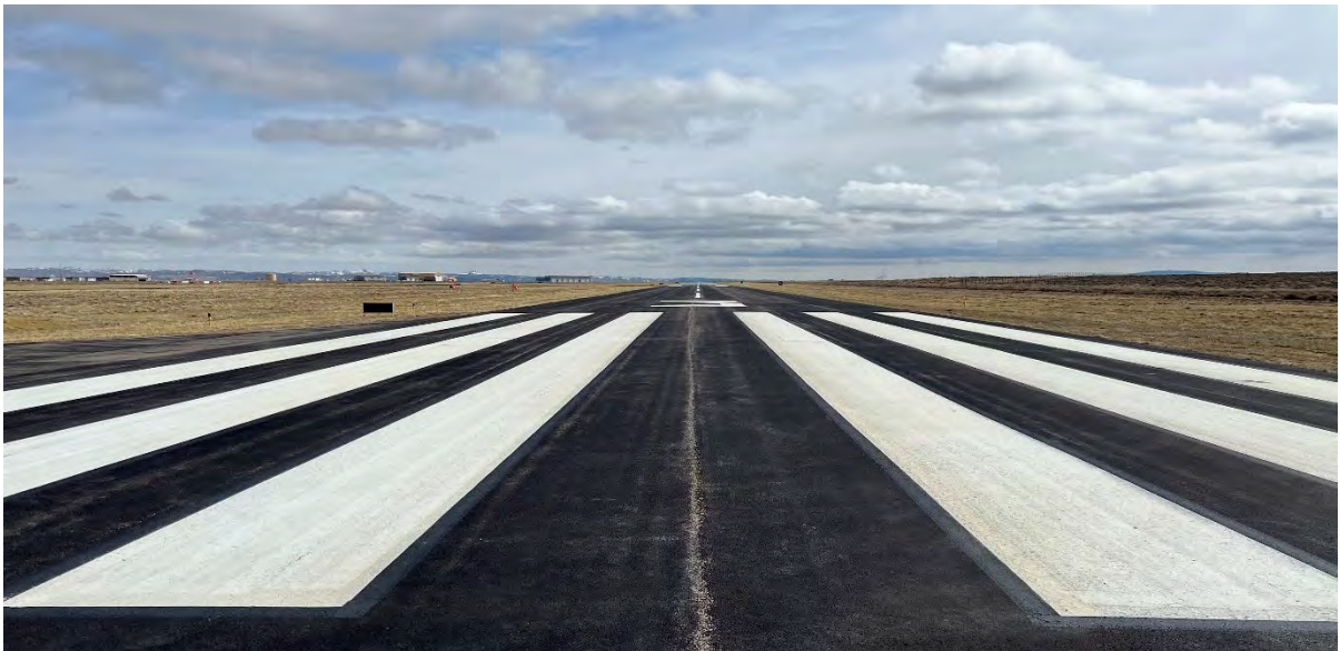
Figure 1-2: South End of Runway 3/21, Looking North
