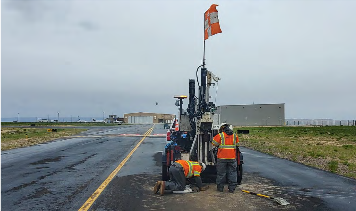
General Site Photo 9: Taxiway C at Boring SW23-321-02, looking Northwest
