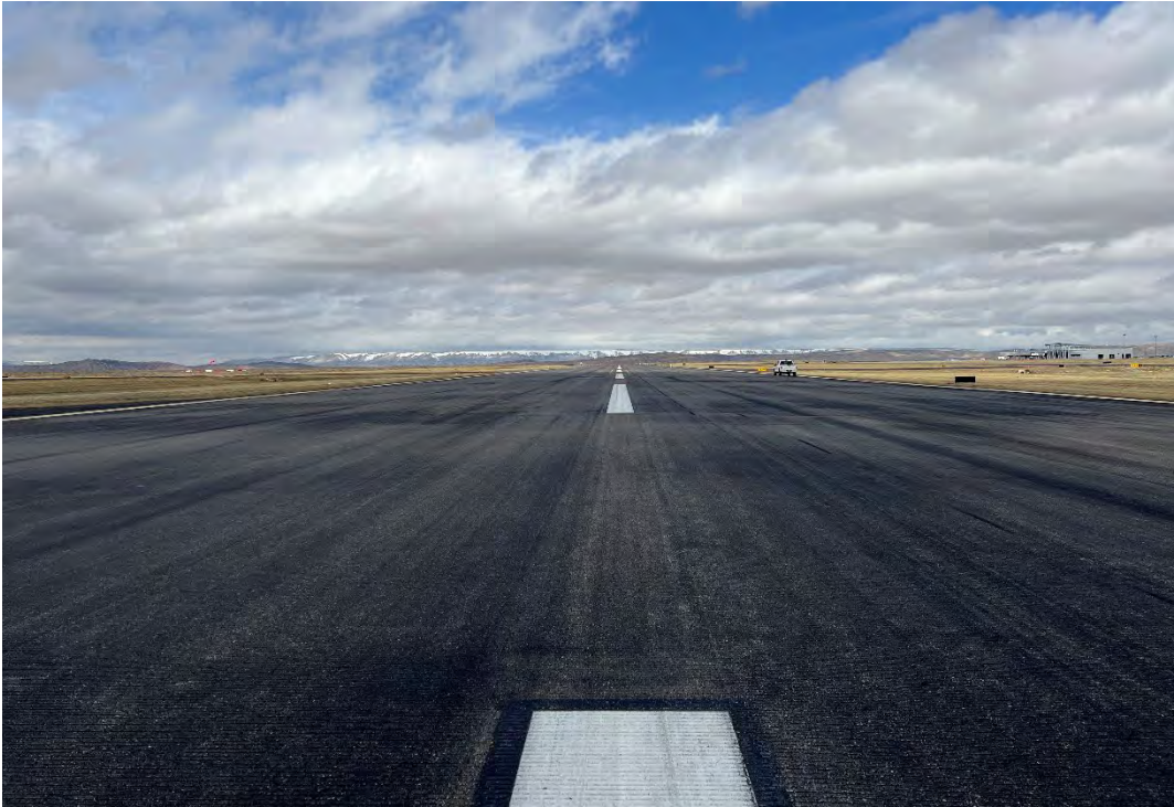
General Site Photo 3: Runway 9/27 at Runway 3/21, Looking West
