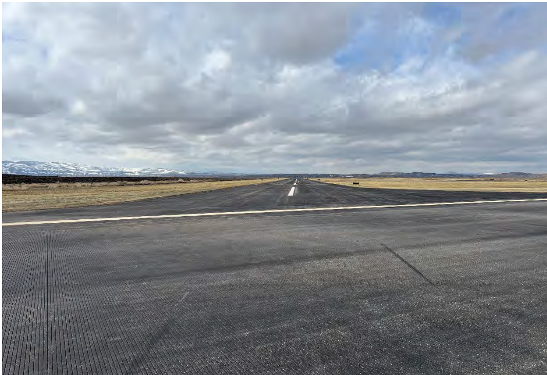
General Site Photo 6: Runway 3/21 at Runway 9/27, Looking Southwest
