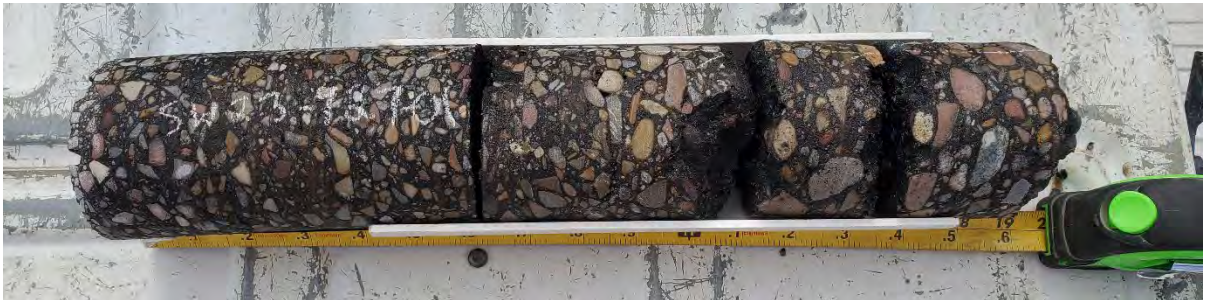
Figure 2-7: Pavement Core Collected at Boring SW23-927-01
